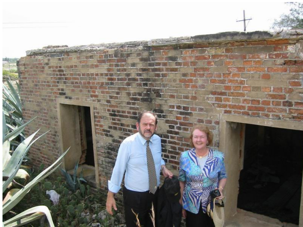
Photo 1 Outside one of the decaying prison buildings in Basuo
